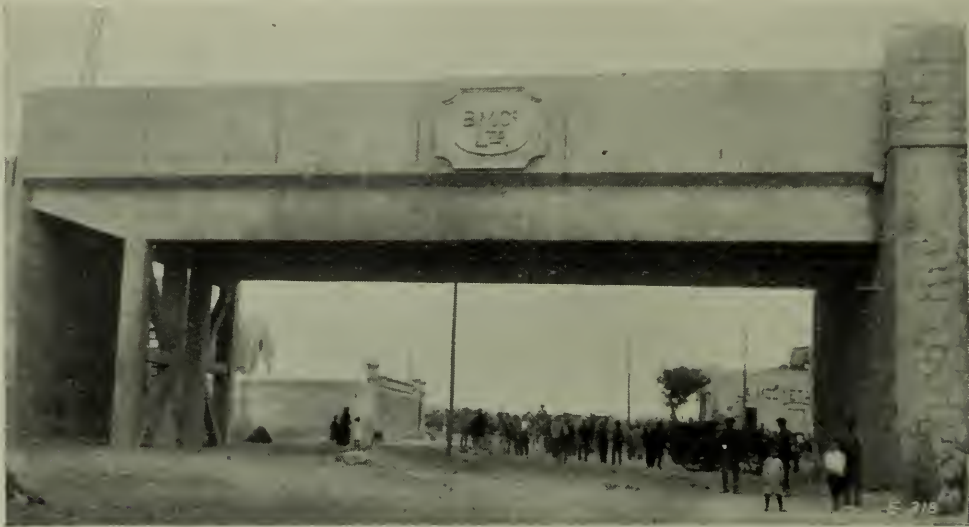
FIG. 2. REINFORCED CONCRETE RAILWAY BRIDGE AT ALMERIA, SPAIN.
